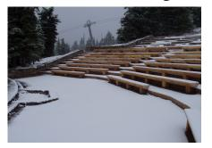
• We had to set post levels in a straight line at the same height. This was critical for a successful project. The benches fastened to square cedar posts with quarter round log risers. The posts had to match precisely to the dado notches in each bench.
